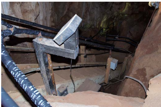
PVC-wrapped handrails in Mercer not only reduce any risk of electrocution, but are also smoother to the touch.
